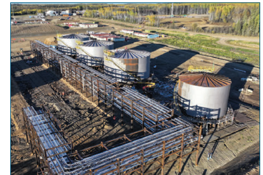
Pipe rack modules
