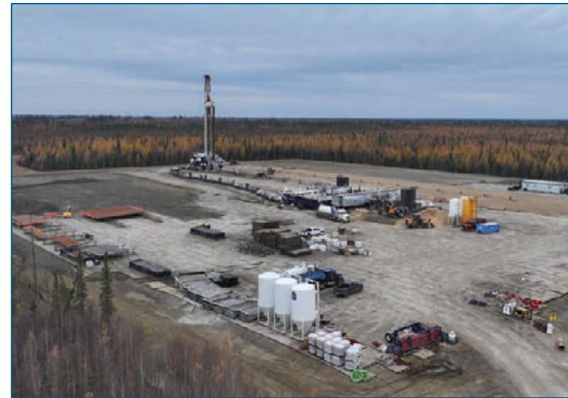
Drilling ongoing (Drilling on Pad A)
