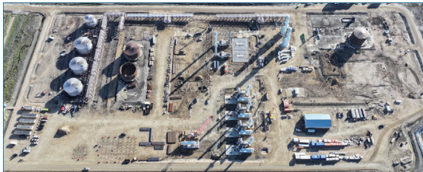
Blackrod Central Processing Facility (CPF)
