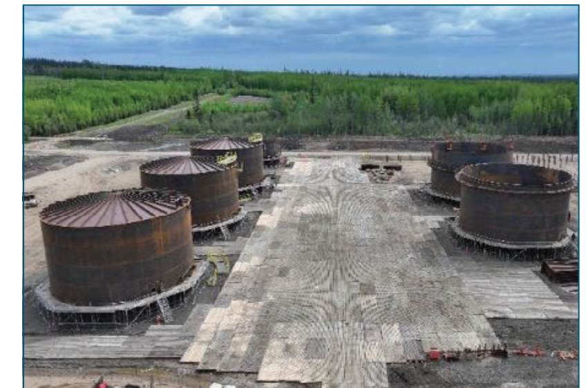
Construction - tank farm
