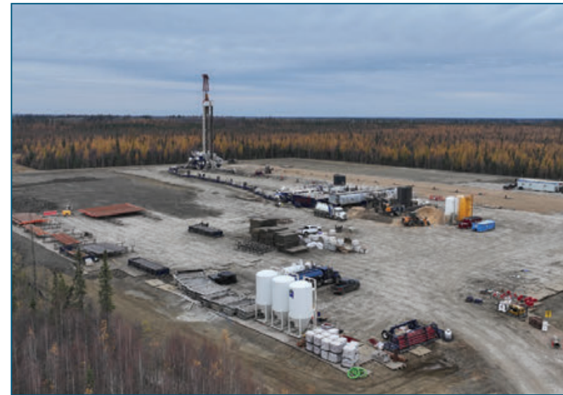
Drilling ongoing (Drilling on Pad A)
