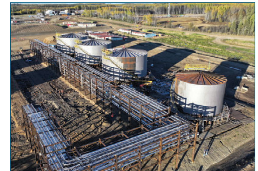
Pipe rack modules
