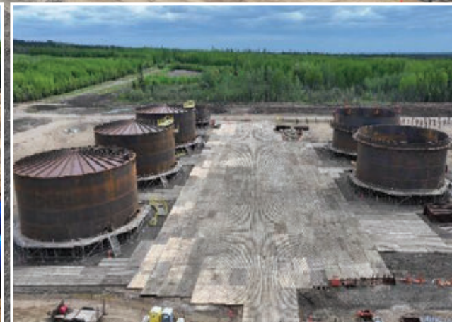
Construction - tank farm
