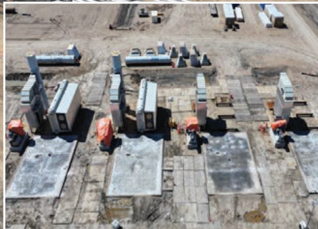
Boiler concrete pads completed
