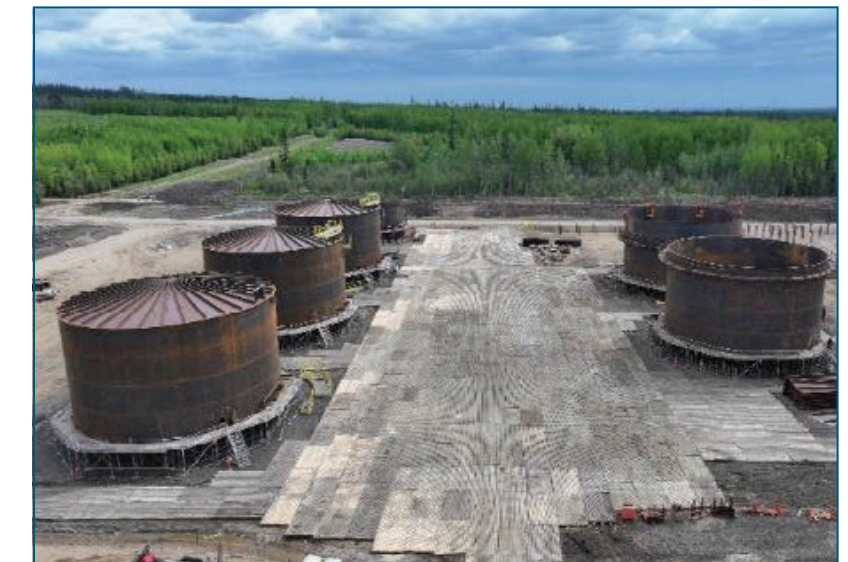
Construction - tank farm
