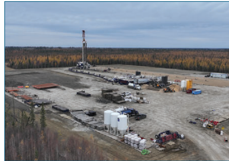
Drilling ongoing (Drilling on Pad A)
