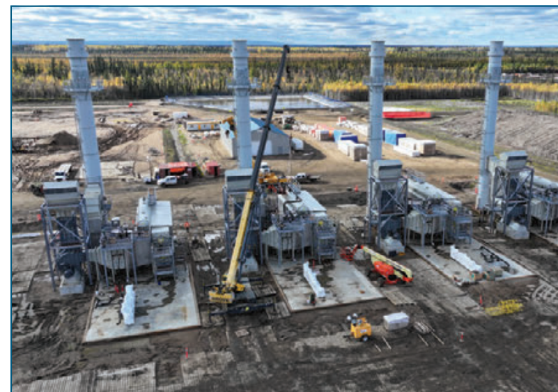
Boilers in place
