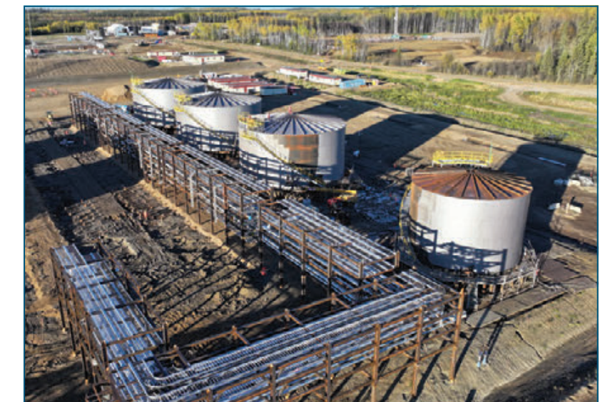
Pipe rack modules
